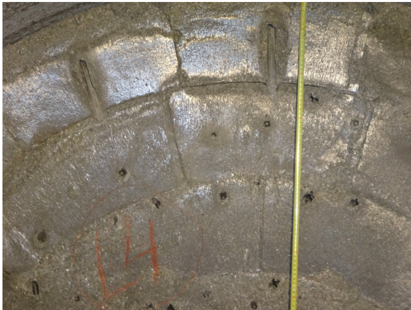
Fig. 57: Waxy aspect of blocks in L4.
