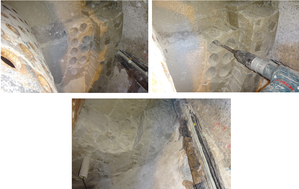
Fig. 59: Extraction sequence of blocks by taking cores.
