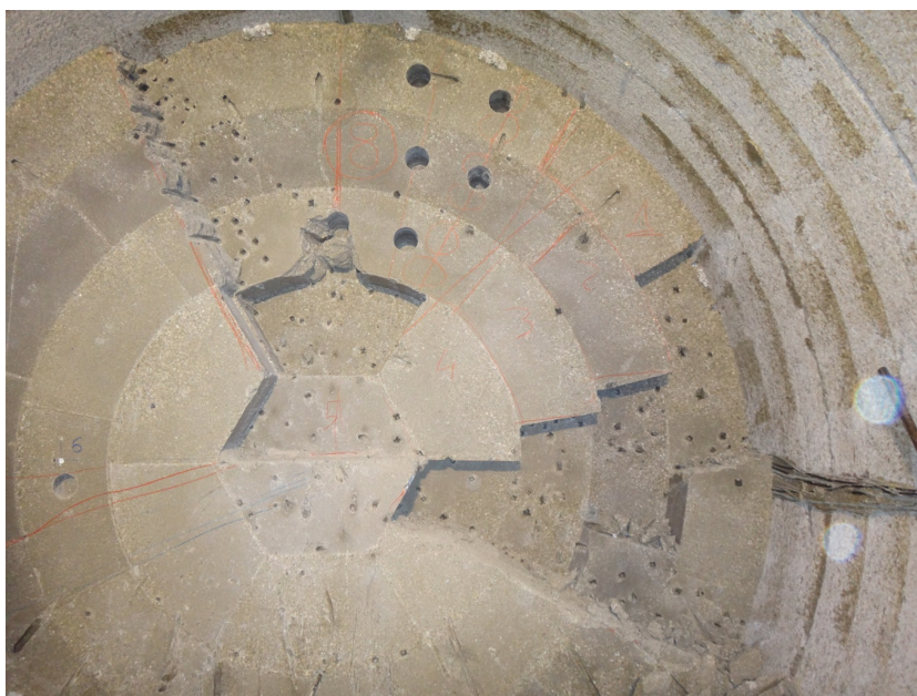
Fig. 69: Partial dismantling of S59.
