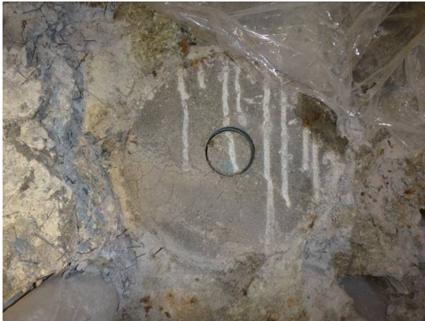
Fig. 31: Emplacement of B-C-36-5 in the interface of PSP-01.
