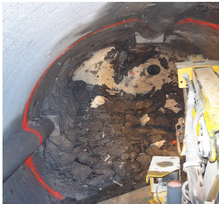
Fig. 20: Marking of plug face on the gallery and left cable duct.
