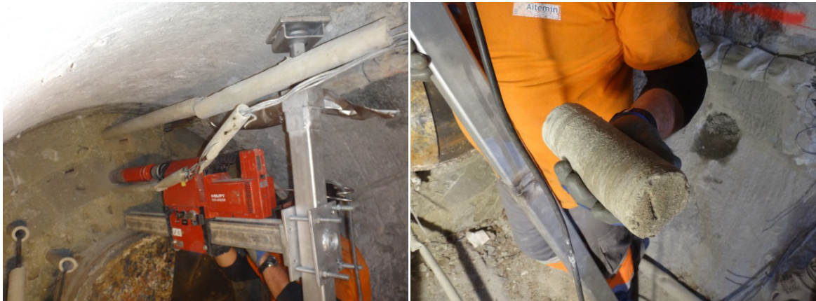
Fig. 43: Details of the bentonite sampling. Drilling machine at the left side and obtained core at the right.
