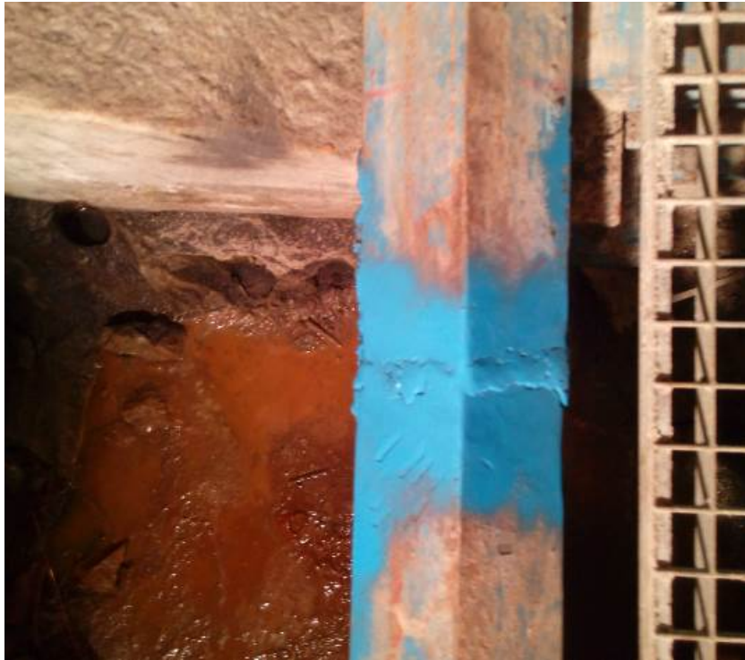
Fig. 10: Detail of welded rail sections.
