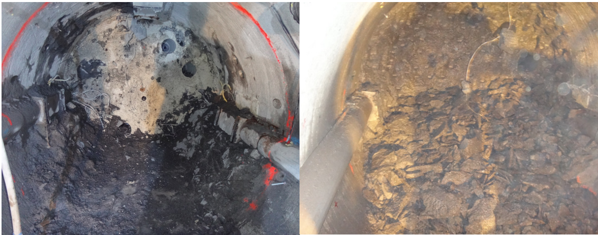
Fig. 21: Detail of the base made with concrete debris in order to facilitate the robot movements.
