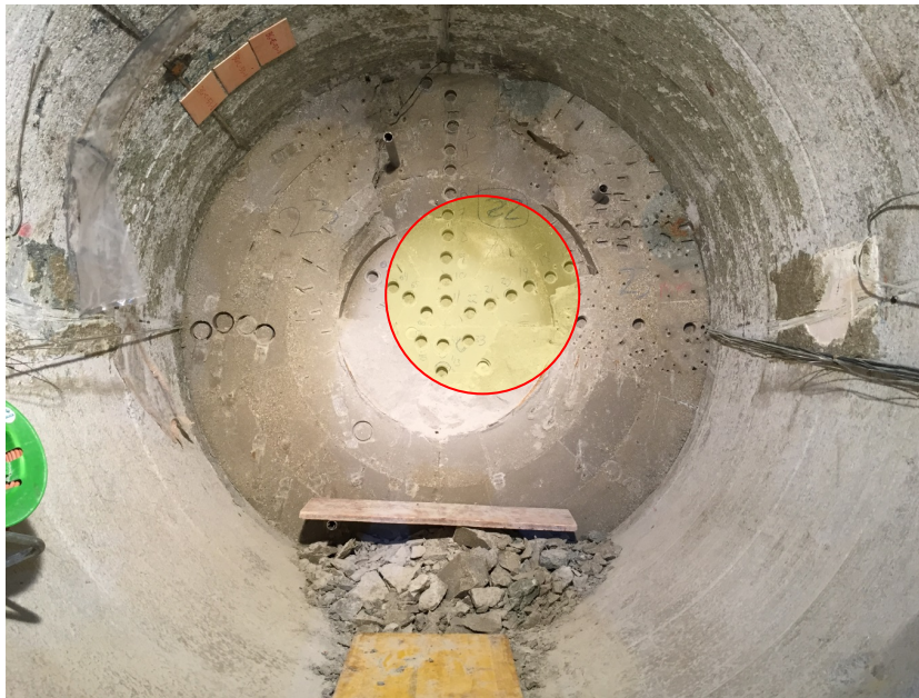
Fig. 55: Protruding bentonite in the centre of the buffer.
