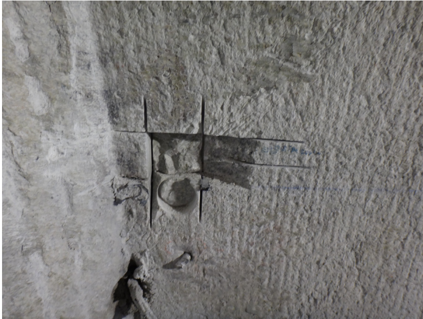
Fig. 70: Granite cut made with radial saw.
