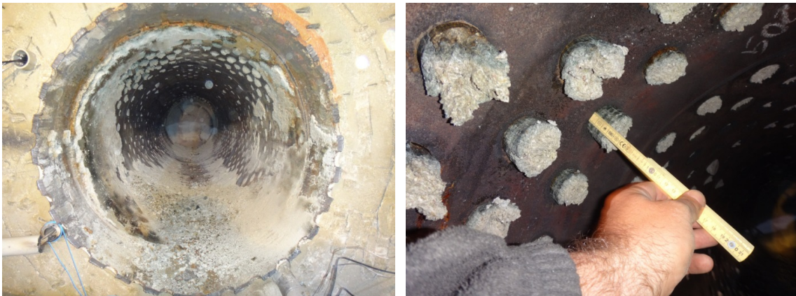
Fig. 51: Inner view of the liner once the heater was extracted (left photo) and detail of the bentonite protrusions inside the liner (right photo).
