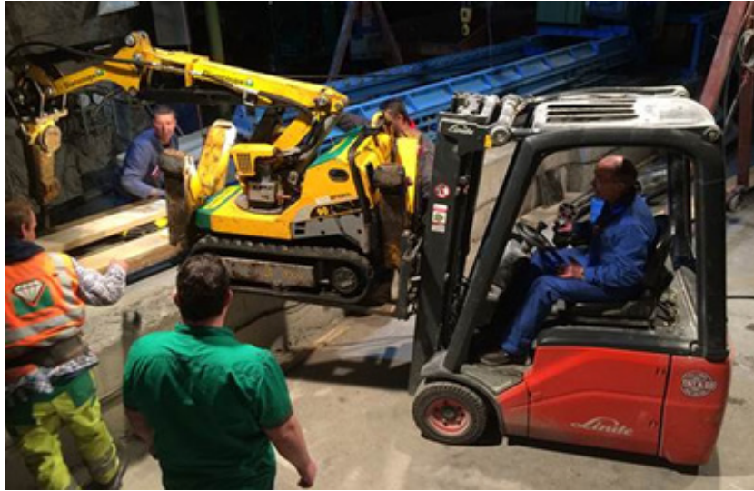
Fig. 19: Robot installation on the drift.
