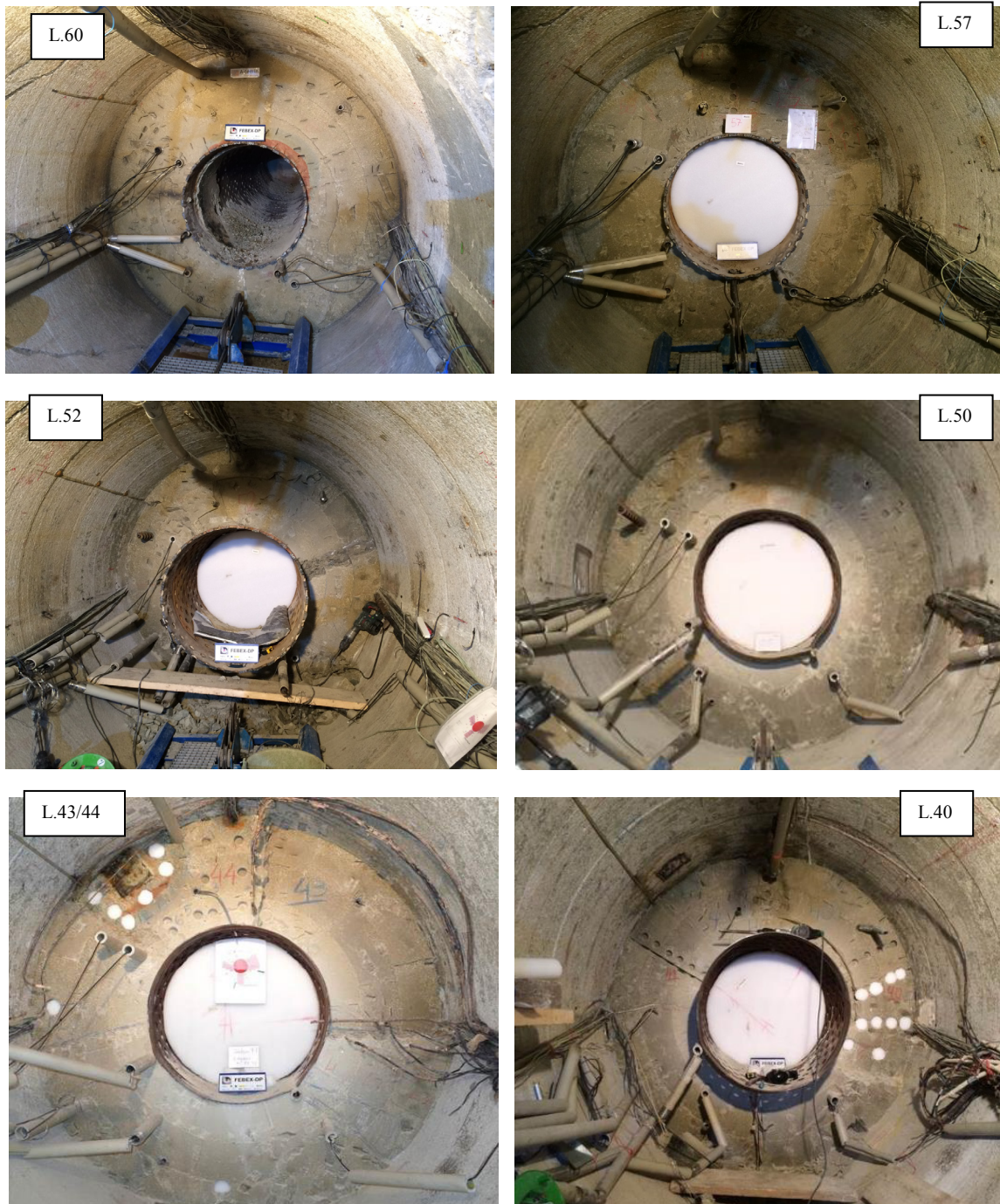
Fig. 54: Sequence of views of the bentonite front from the heater #2 front to the end of the gallery.
