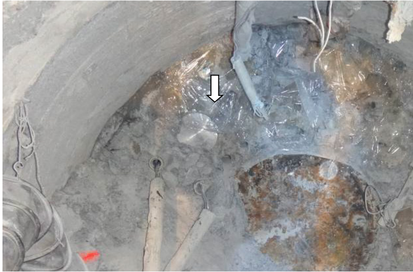
Fig. 30: View of PSP-01 before removal.
