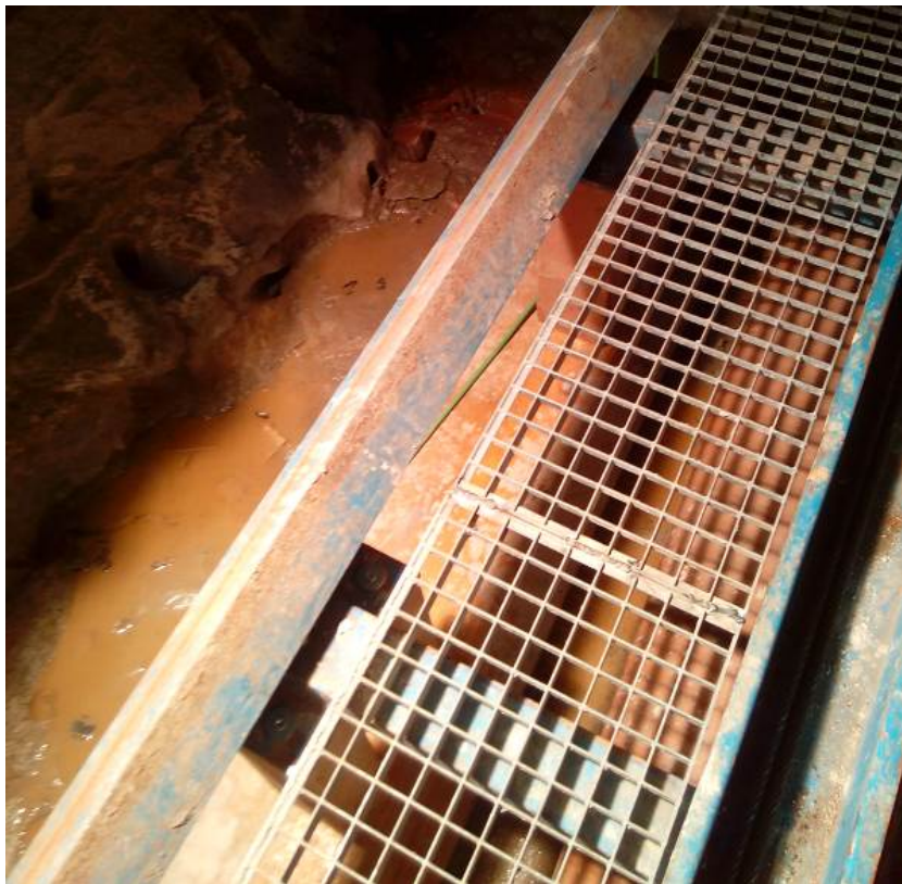
Fig. 9: Detail of wooden feet and pathway on the newly installed tracks.
