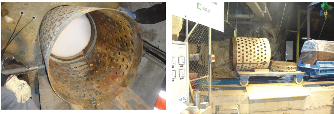
Fig. 53: Dismantling of a liner section.
