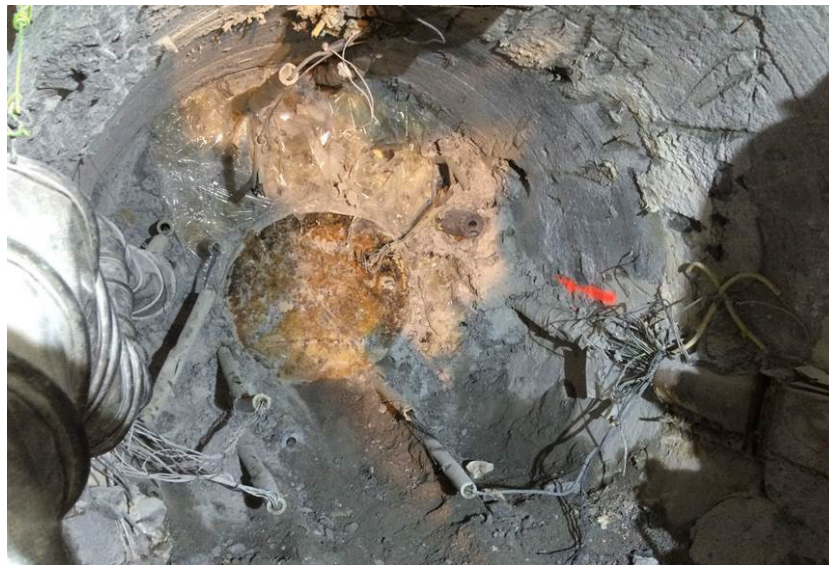
Fig. 29: Plug dismantled and dummy face exposed.
