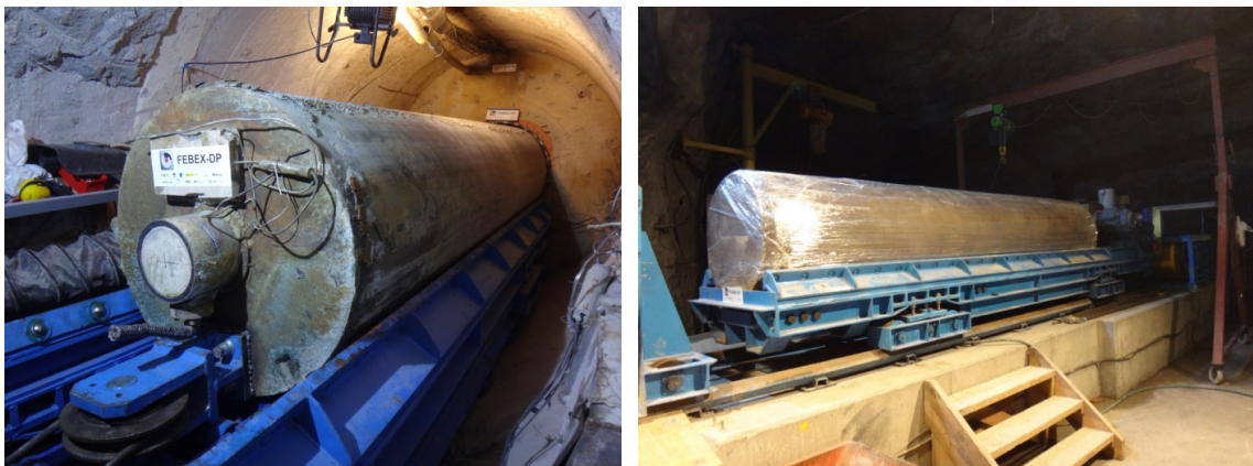
Fig. 49: Extraction of heater #2 (at the left) and general view of the heater at the drift entry (at the right).
