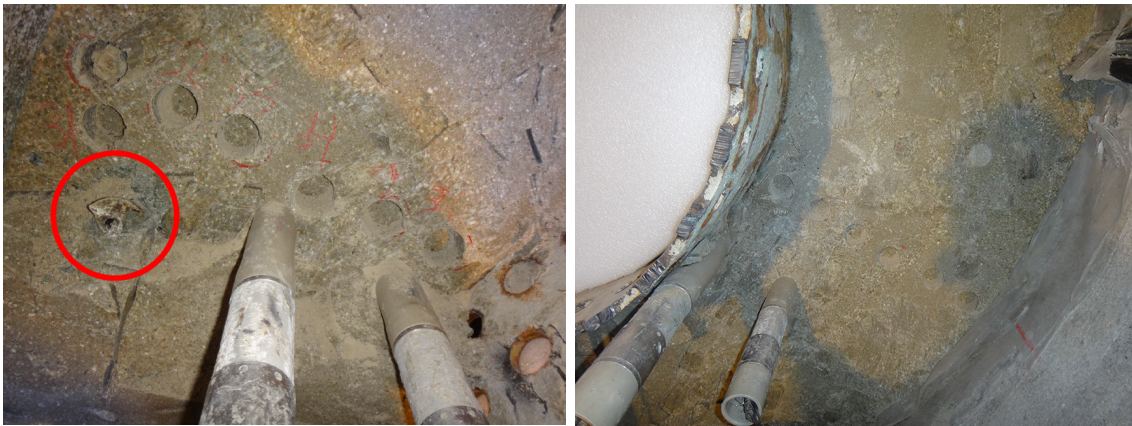
Fig. 39: Upper left part of the barrier showing the pipes and the corrosion halo around an abandoned drill bit (left) and lower right part of the barrier with the plastic sheet between granite and bentonite (right).
