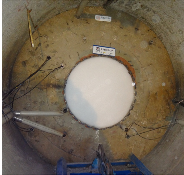
Fig. 125: EPS plug placed at the front of the liner once the heater was extracted.
