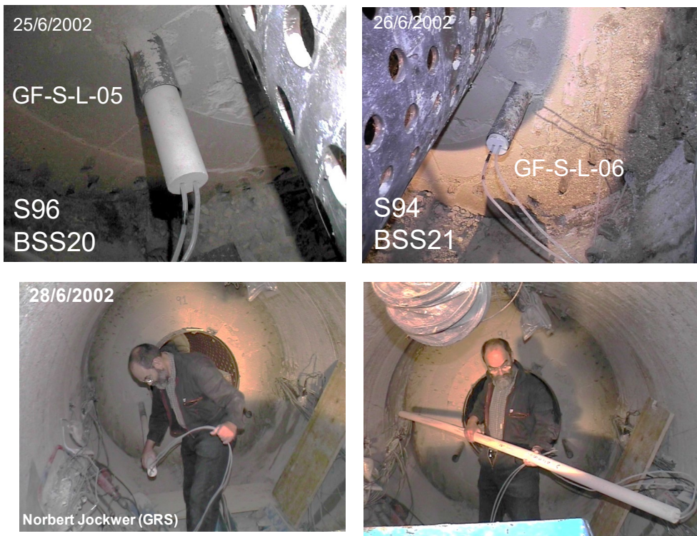
Fig. E-5: Visual aspect of the GRS pipes GF-S-L-05 (left side, bentonite Section 96 (BSS20): 25 June 2002) and GF-S-L-06 (right side, bentonite Section 94 (BSS21): 26 June 2002) during dismantling operations of the Heater #1
