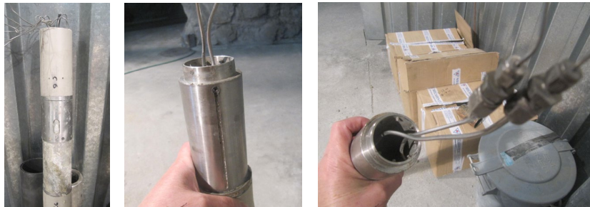
Fig. 32: Fluid sampling element and rod: a) after dismantling, b) element without the porous 316L stainless steel sintered filter, and c) detail of the 1/8 to 1/16" tube reduction Photo taken during dismantling activities in 2015.
